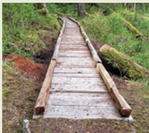
AFTER: WTA volunteers cleared 6 miles of downed logs from the Downey Creek Trail, including the repair of this puncheon, using materials found on site. Photos by Mark Huston
