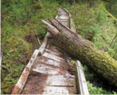
BEFORE: Fallen logs had taken their toll on the Downey Creek Trail, including this puncheon bridge through a wet area.
